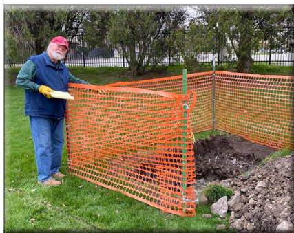
Bernie Ashyk inspecting phase 1 of new water line for the club.
